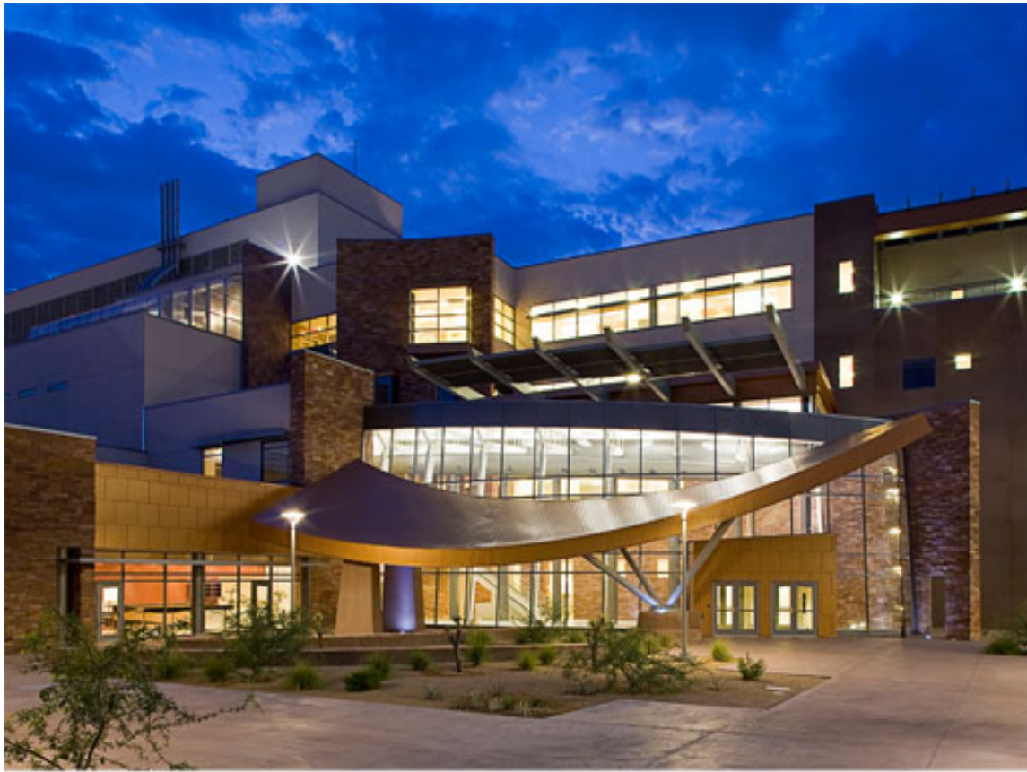
UNLV Science, Engineering & Technology Building - Las Vegas, NV
